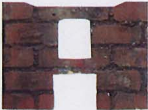
Decorative masonry-like panels
